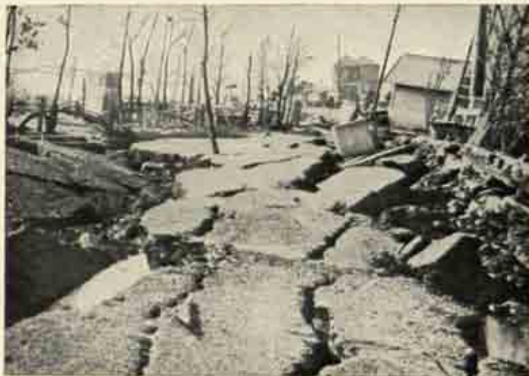
(A) Gaping fissures in a country road near Yokohama
